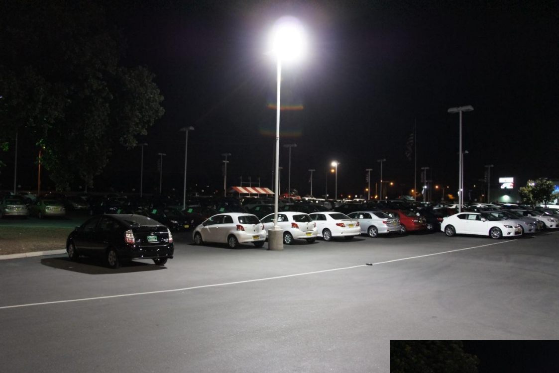
BEFORE 1077 Watt Metal Halide
